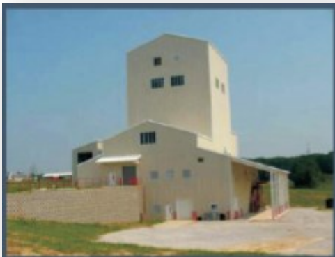
NCSU Feed Mill
